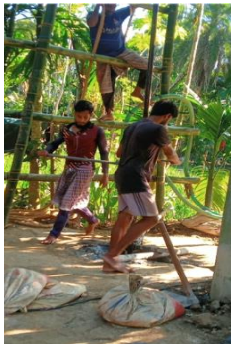
Installing a tube well for pure drinking water
